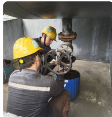
Repair team installing
